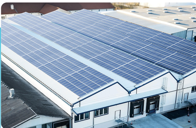
Industrial Rooftop Solar Installation
