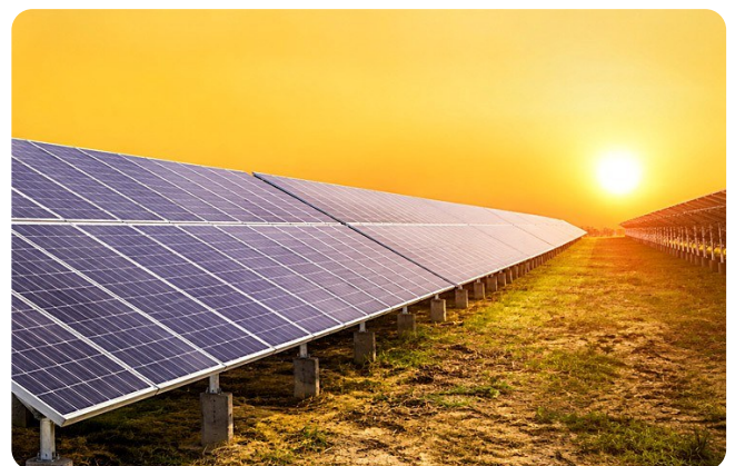
Ground-Mounted Solar Installation
